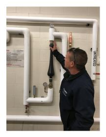
**Go with the flow** -- The water needs to enter the REALice system at the wide part of the venturi and exit through the small end to treat the water
