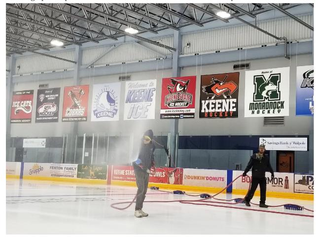
The **Blue** adaptor creates a narrow mist that diffuses the water to create a clear, durable ice surface.
